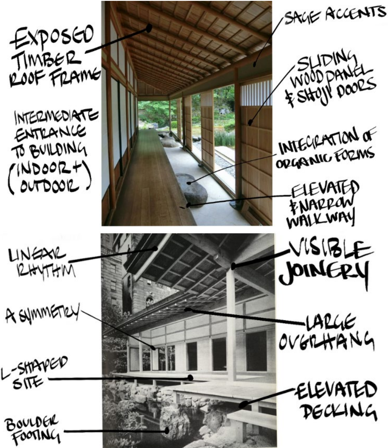
Precedent study of Japanese porch typologies and joinery-based construction techniques shaping thresholds, shelter, and detail. Historic Precedent Study —————
